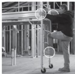
When you are on the plank, always keep your body within the footprint or outline of the board. Do not overreach or stand on anything else other than the plywood deck. If the job is too high, you probably need to add height to the scaffold. When loading equipment or materials onto the scaffold, do it slowly and carefully to prevent tipping and distribute them evenly. When using guardrails, be sure to close and latch the gate.
