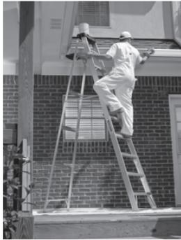
Position stepladders and other self-supporting ladders so that all four legs are on solid, level ground. Lock the spreaders in the fully open position.
